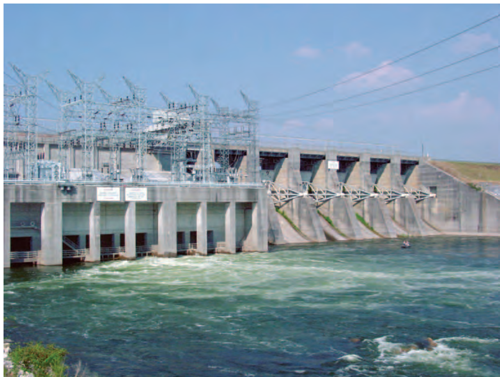
Figure 11.1 Hydroelectric generating facility. (Courtesy of Mark Nelms)
