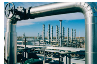
▲ Aluminum is stable because its oxide forms a protective film over the underlying metal, preventing further oxidation.
