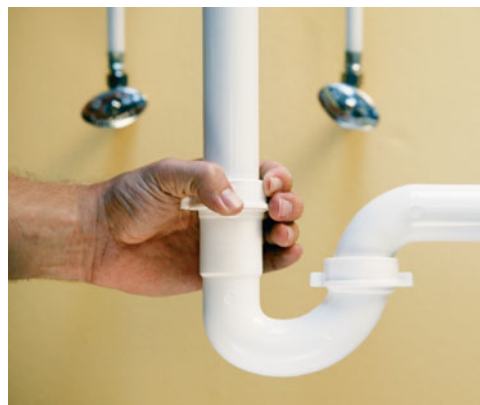
► FIGURE 20.15 Polyvinyl Chloride Polyvinyl chloride is used for many plastic plumbing supplies, such as pipes and connectors.
