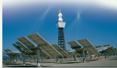
Solar power tower
